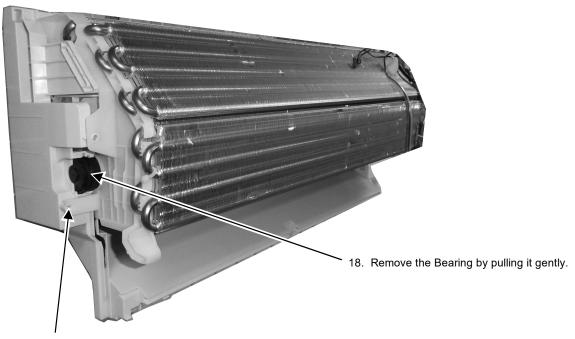
17. Remove the screw from the Evaporator.
