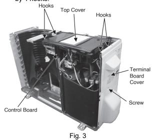
5 Remove the Control Board as follows:
