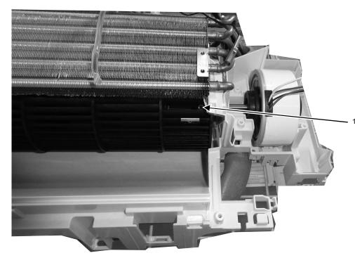
16. Remove the screw that holding the Cross Flow Fan and Fan Motor axis.
